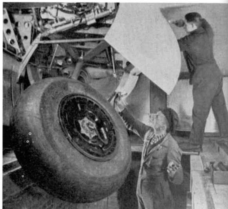
ABOVE: A Ju 88 undergoes an undercarriage retraction test at the factory and shows the main-wheel rotating into its housing behind the engine, under the watchful eye of a technician.
