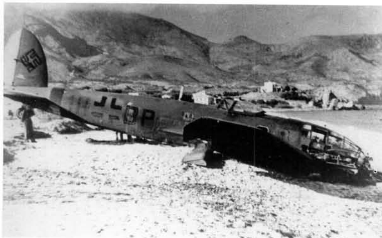
BELOW: This He 111 from 6./KG 26, coded 1H+BP, made an emergency landing on the Spanish coast. Note that the usual white outline to the fuselage cross, swastika and the fuselage band have been overpainted in black for night operations.
