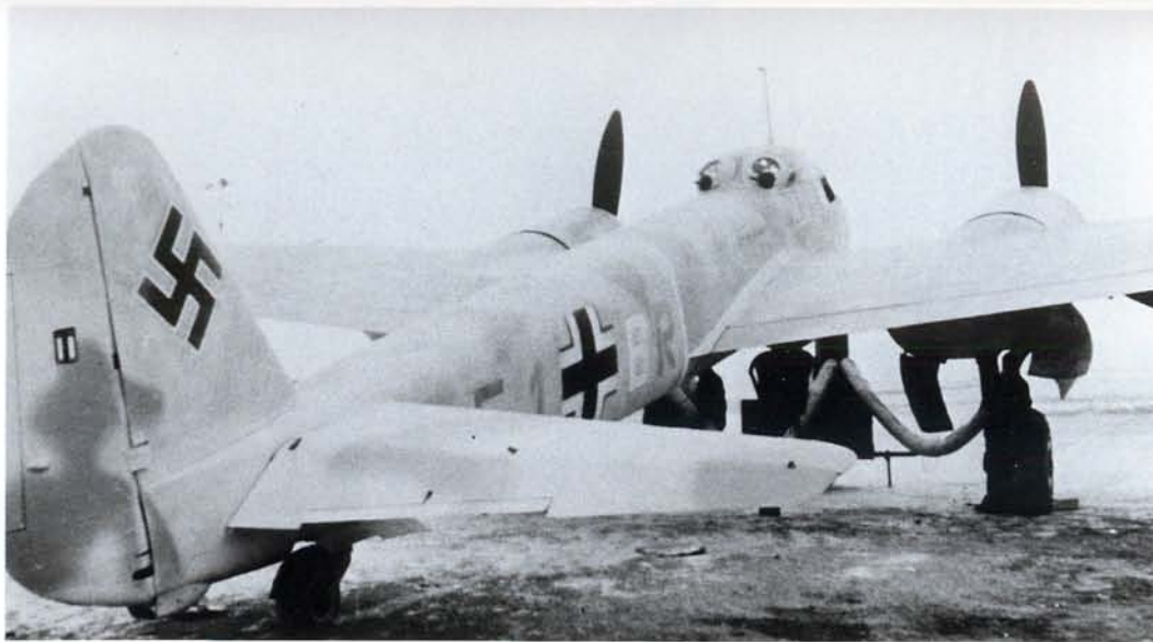
LEFT: A Ju 88 of 7./KG 76 on the Eastern Front in the winter of 1941-1942. The aircraft wears an unusual toned down colour scheme with white paint oversprayed on the standard green camouflage. Seen at the front of the aircraft are the pipes from the combustion heater unit.
