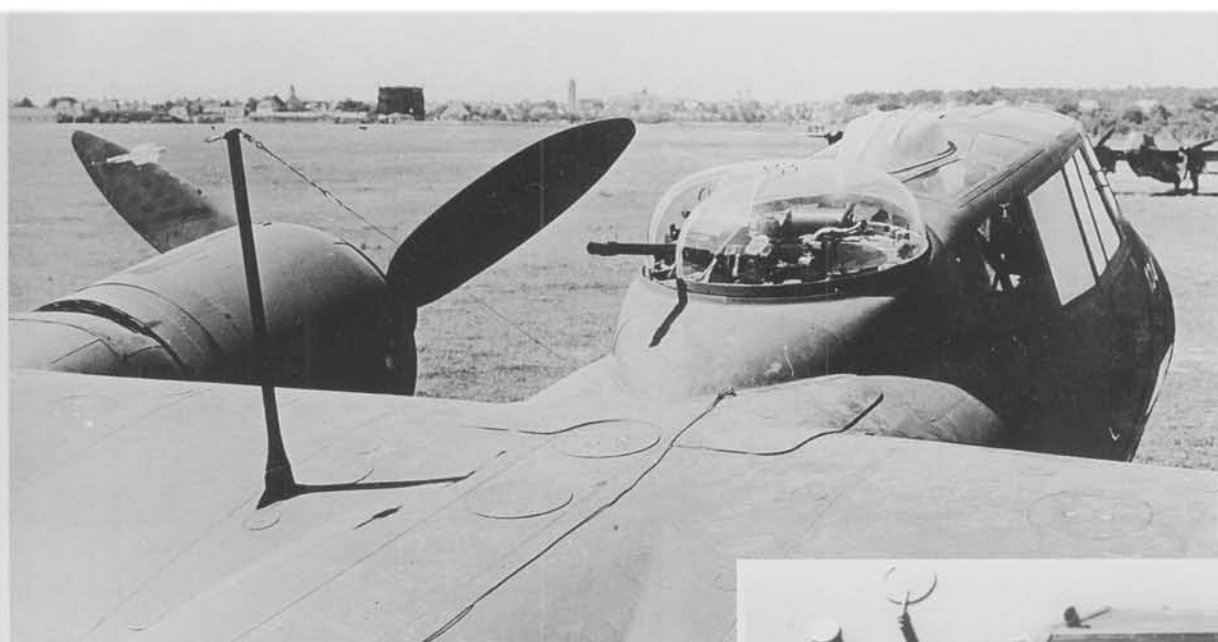
LEFT: A close-up of the Do 217 E-2, showing the electrically-powered dorsal turret with a single 13 mm MG 131 machine gun.
