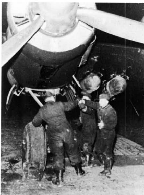
RIGHT: Ground crew crank the inertia starter handle to start the starboard engine of a Ju 88 of KG 1, before it sets out on a night attack.
