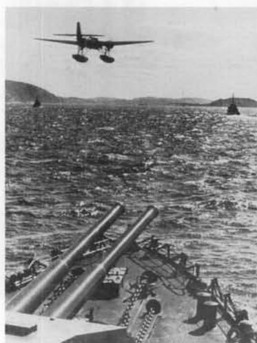
ABOVE: A Heinkel He 115 floatplane passes low over German warships during an exercise. Although the aircraft was robust and reliable, its low maximum speed of 290 km/h (180 mph) at sea-level restricted its use in its intended role of torpedo-bomber. In service, the main roles it performed were those of minelaying and maritime reconnaissance.
