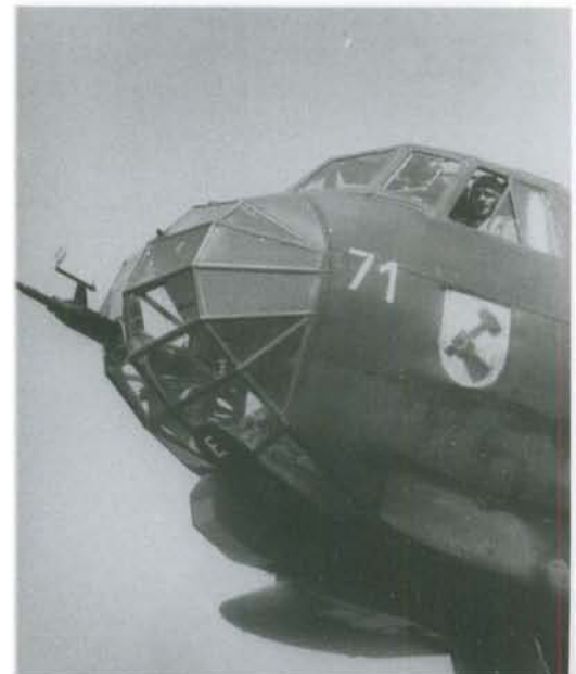
RIGHT: A Do 217 E in this photograph shows the 'Holzhammer' emblem on the port side and also has an MG FF cannon fitted in the nose.
