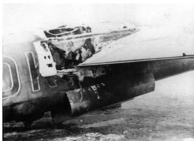
LEFT AND BELOW: The He 177 was rushed into production, and many were lost following engine fires. All attempts to introduce the aircraft into combat between the beginning of 1942 and September 1943 ended in failure. The type was withdrawn for a major programme of modifications. This He 177 A-1 was being used as a trainer with Flugzeugführerschule (B) 16 at Burg/Magdeburg with many of the unit's aircraft ending up this way due to technical malfunction.
