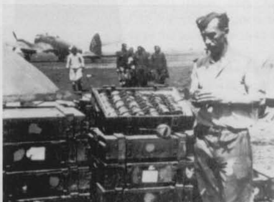
ABOVE: The SD-2 anti-personnel bomb weighed 2 kg (4.4 lbs), and was dropped in a container as a cluster munition. The photograph shows the weapon in the folded, safe position. while ABOVE RIGHT An armourer inspects a newly delivered consignment of SD-2 bombs.
