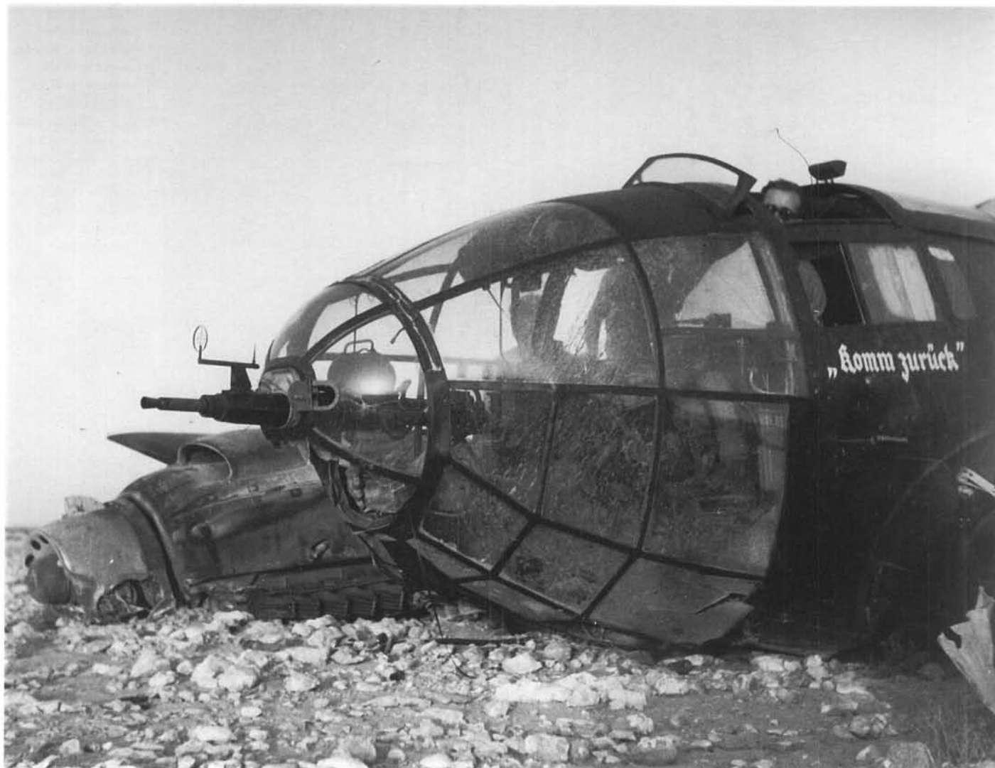
ABOVE AND BELOW: This He 111 H-6, W.Nr. 7094 coded 6N+FH from I./KG 100 was brought down in North Africa. The inscription below the pilot cockpit reads "komm zurück" ("come back") which did not bring this crew any luck. Note the rear view mirror fitted to the front of the pilot's sliding hatch.
